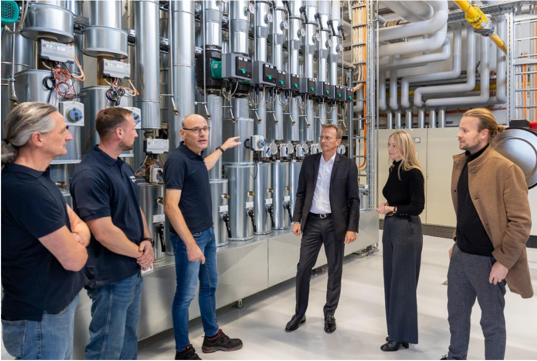
Flender uses the waste heat from the company's own hardening shop to heat its site in Bocholt, thereby saving significant amounts of gas and CO 2 emissions.
